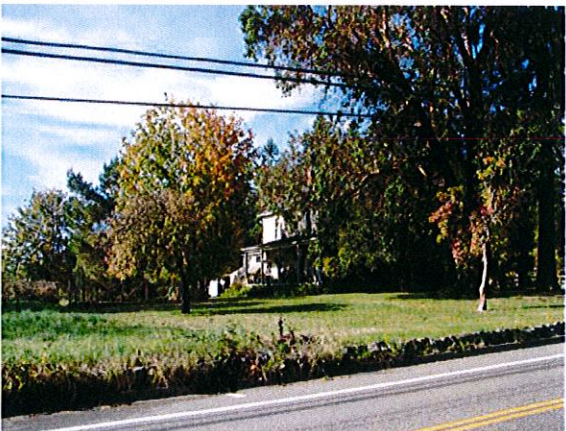
EXISTING CONDITIONS ALONG FERNCLIFF AVE
