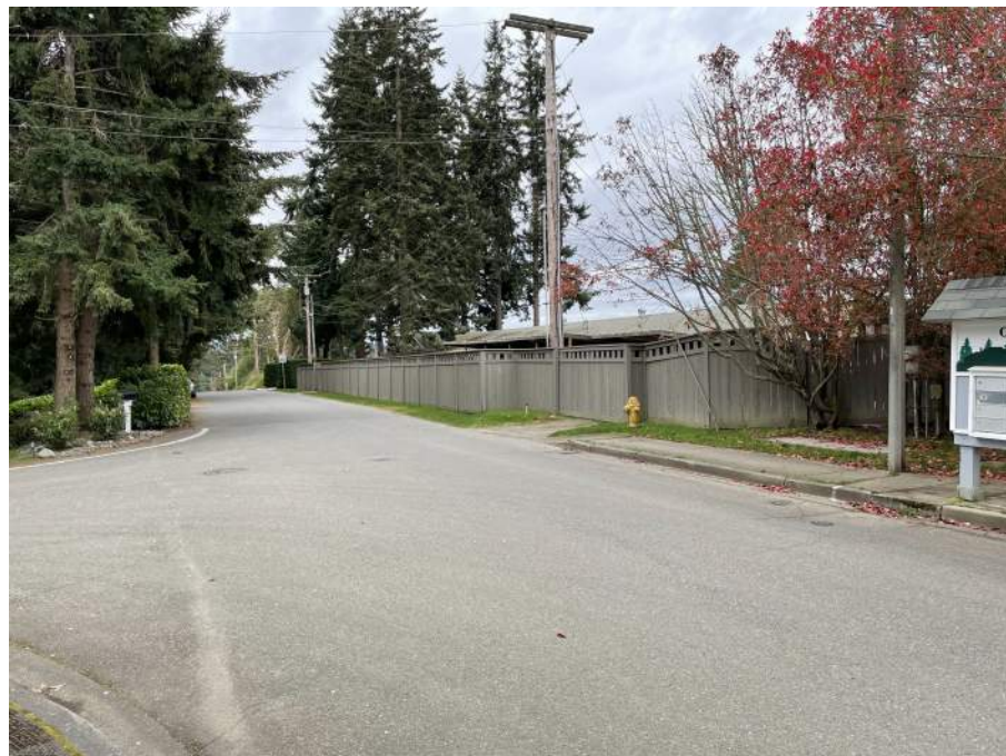
CHERRY AVE LOOKING SOUTH AT SERVICE ENTRANCE
