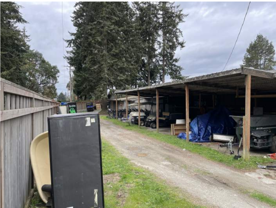
SERVICE AREA ON EAST SIDE OF SERVICE SHED
