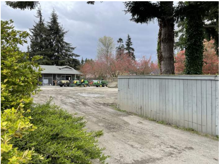
SERVICE YARD AT MAINTENANCE BUILDING
