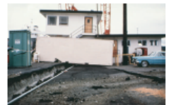
Photograph showing the damage to a building caused by liquefaction during the 1994 Northridge earthquake. The building is a multi-story structure that has been severely damaged, with significant structural failure and debris.
