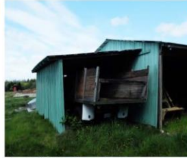
Fig. 15b. End bay storage.
