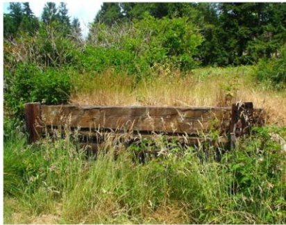
Fig. 16a. Suyematsu loading dock.
