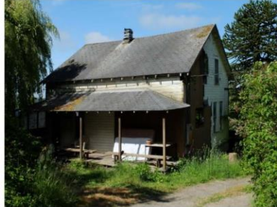
Fig. 8b. NW elevation with mixed siding.
