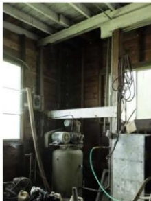
Fig. 10e. NW shed corner.
