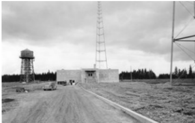
Battle Point Transmitter Station
