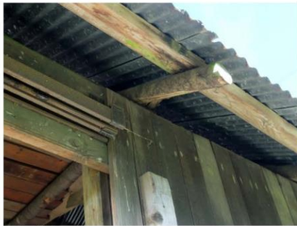
Fig. 9d. Pole rafters and corrugated roof.
