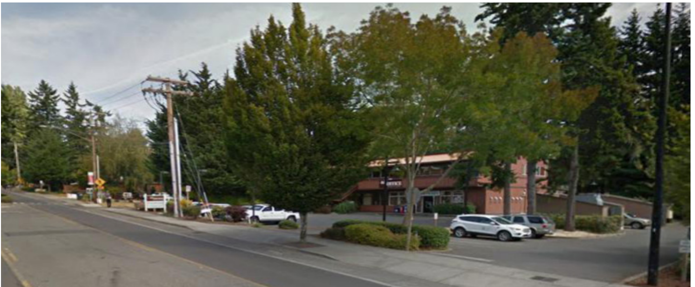
Figure 33: Madison Ave N Looking North with Center Turn Lane and Multiple Curb Cuts
