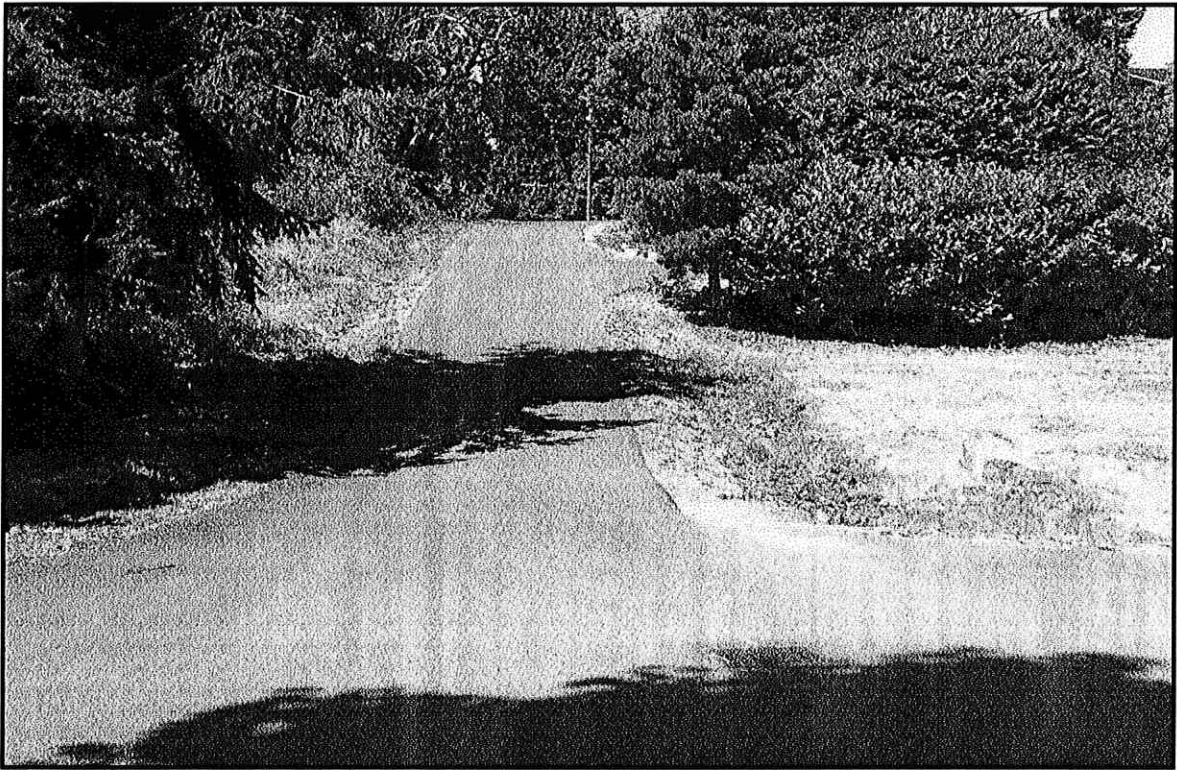
A view of the Mountain View Road NE facing northwest with the subject on the right.
