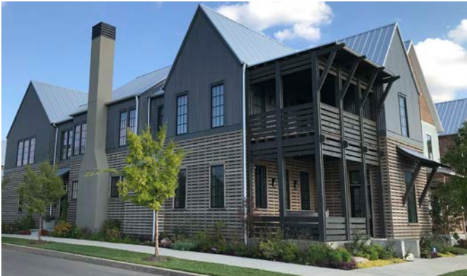
Example of an Engaged Porch
