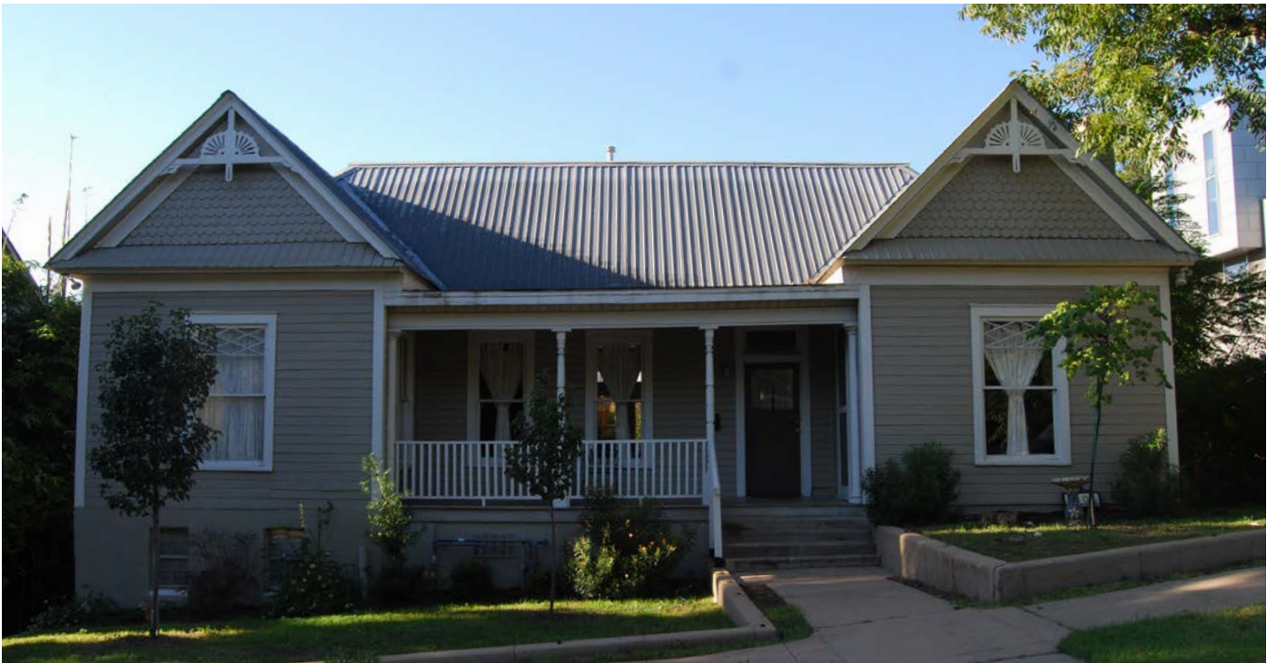
Example of an Engaged Porch
