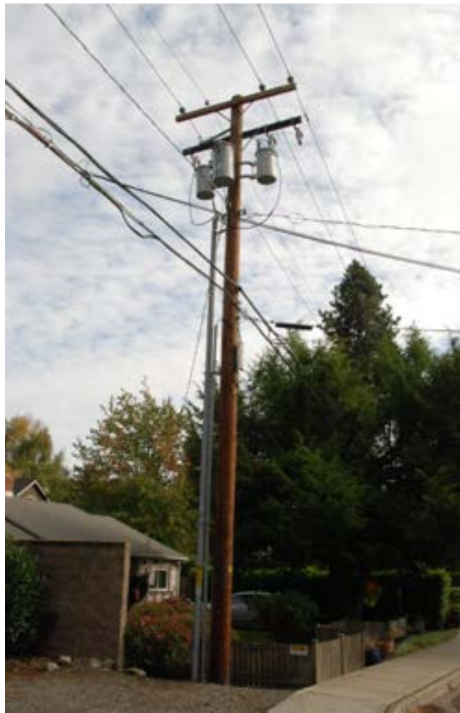
Typical Three Phase Distribution with Three Phase Transformer Bank (with underground service connections)
