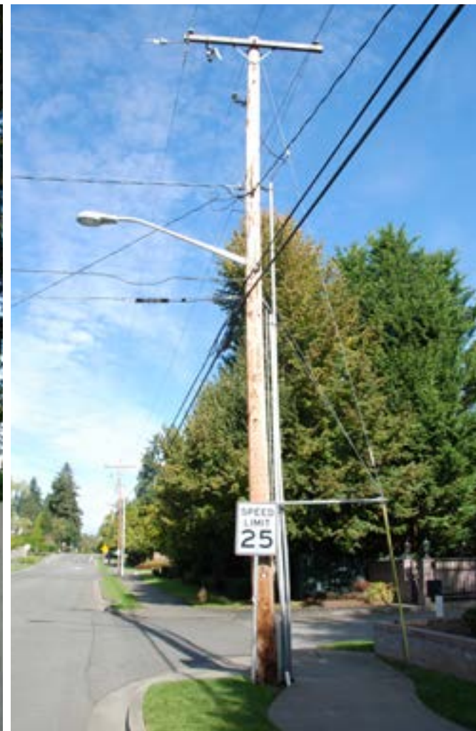
Typical Three Phase Distribution with Sidewalk Guys & Anchor
