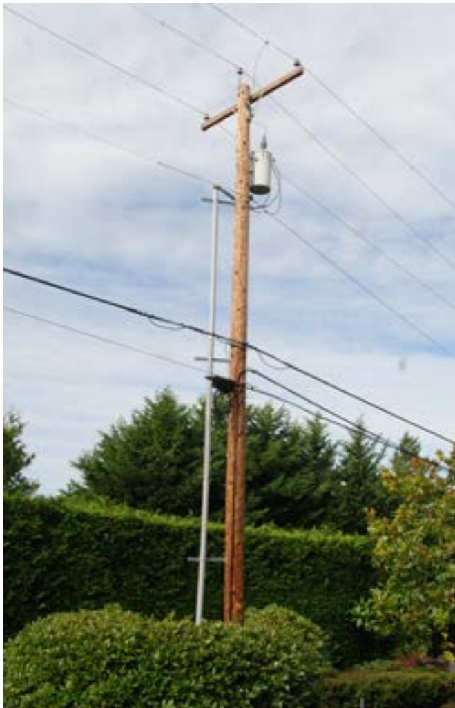
Typical Three Phase Distribution on Cross-arm (with single phase transformer and underground service connection)
