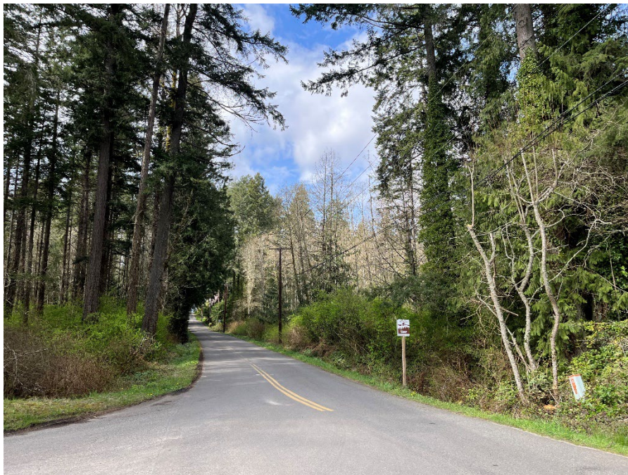
Exhibit 2. An aerial distribution line along NE Bergman Road.
