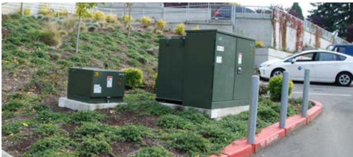
Three phase pad-mount transformers often serve a single commercial customer (but may serve multiple customers) and may be pair with single phase transformers in response to particular service needs
