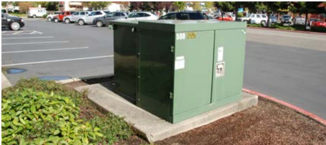
Typical Underground Distribution Three Phase Pad-mount Transformer (5' X 5' X 5' typical but can vary by transformer output rating)
