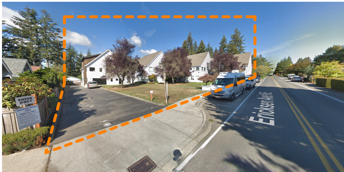
VIEW FROM SOUTH APPROACH
