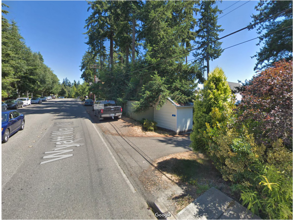
WYATT WAY NE - LOOKING EAST
