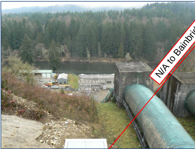
Figure 5-8: Centralia Power Canal penstock, 208 feet above Nisqually River.
