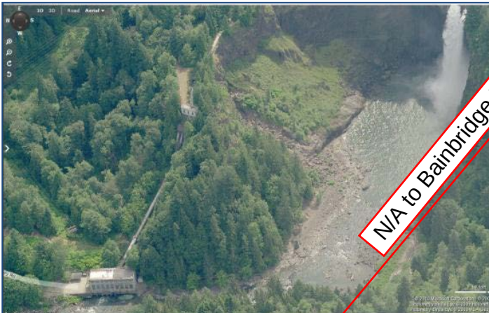
Figure 5-5: Penstock below Snoqualmie Falls.
