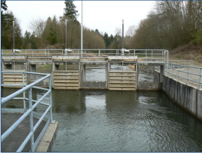
Figure 5-7: Water intake structure with flume (Power Canal) in the background.
