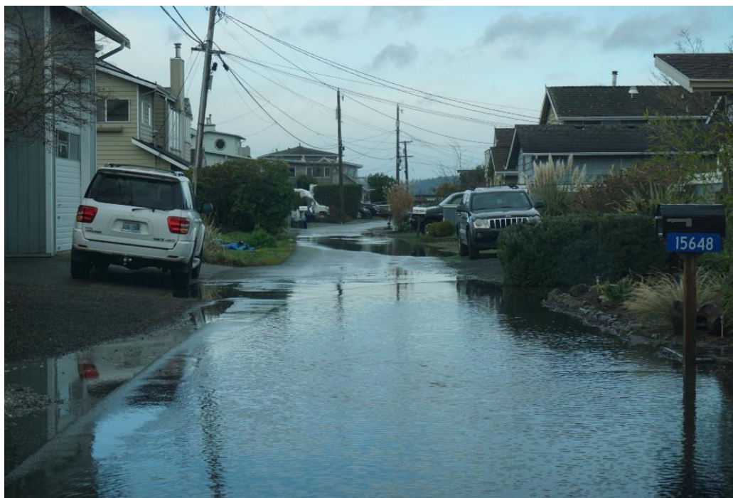
Figure 15: Point Monroe Drive
