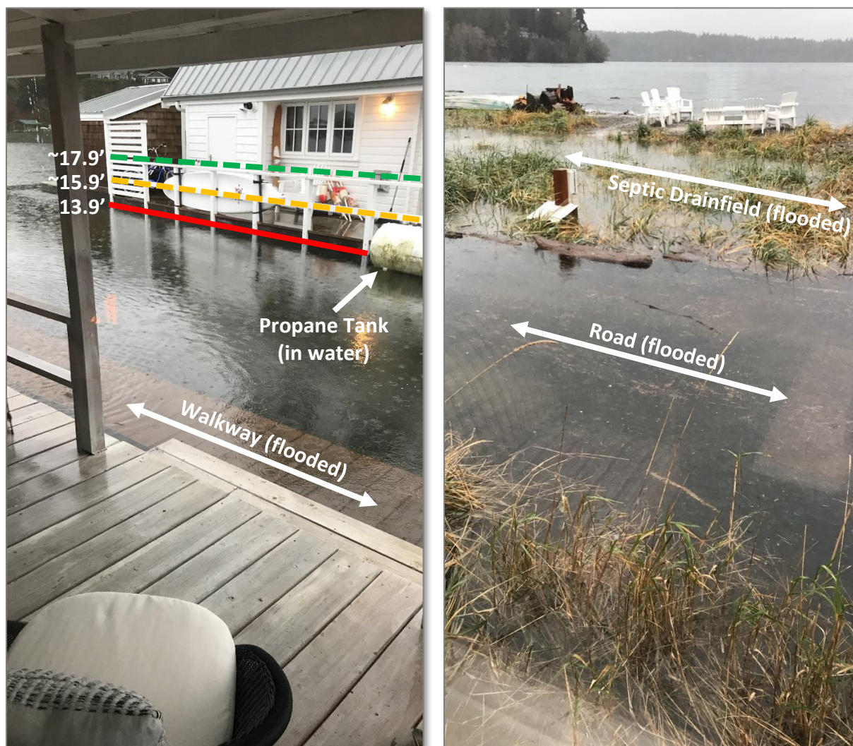
Figure 2. January 4, 2021 “King Tide” Flooding on Bainbridge Island
