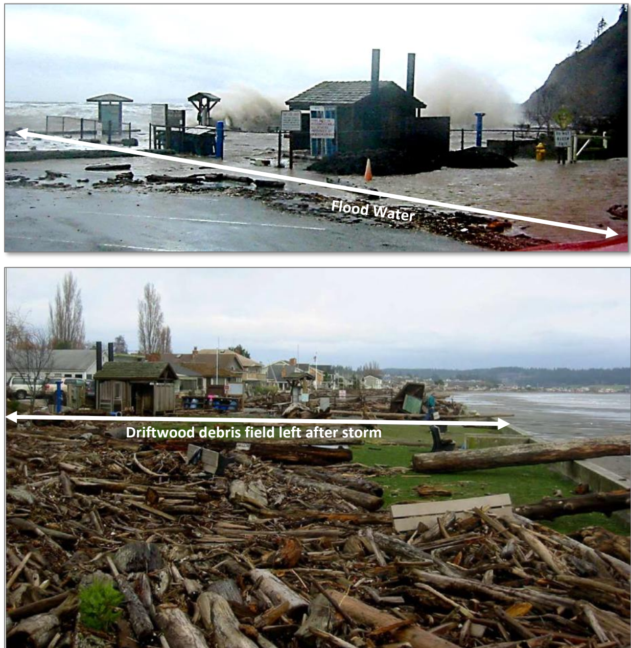
Figure 3. February 4, 2006 King Tide Flooding and Damage
