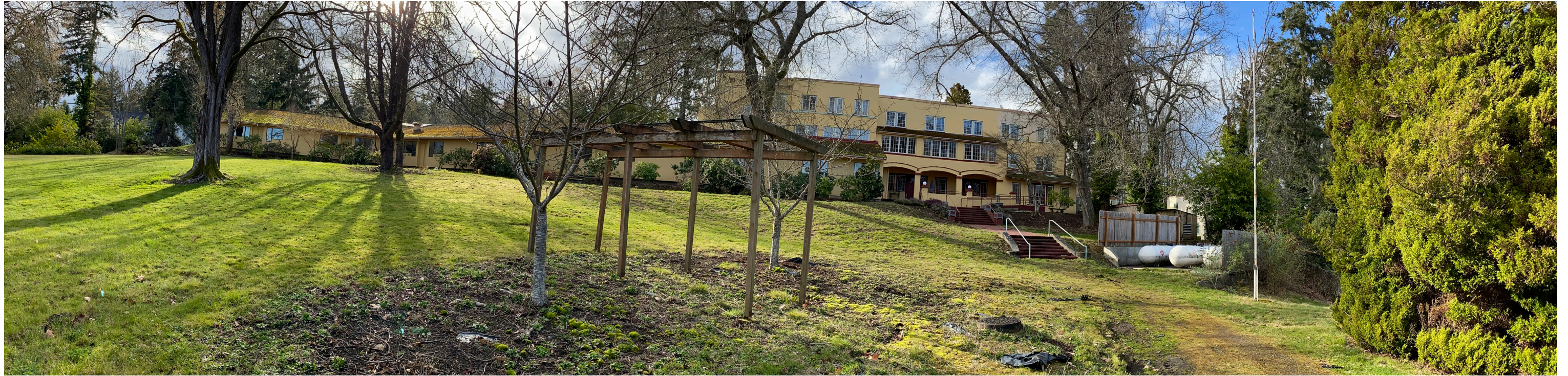
VIEW FROM MANITOU BLVD
