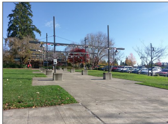
Figure 2 – Town Square Structure
