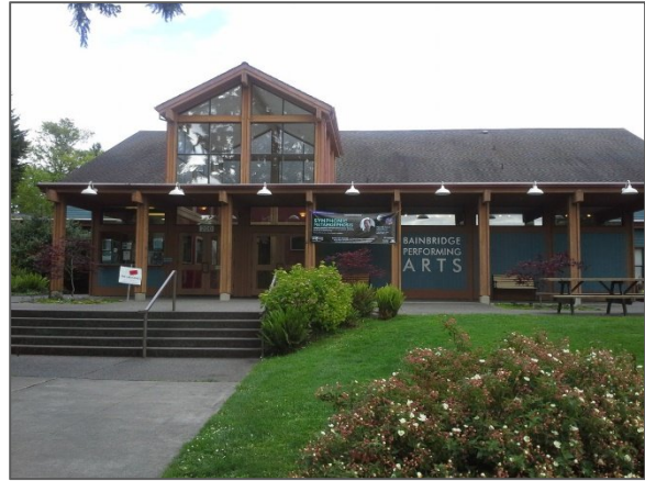
Figure 6 – Existing BPA Building
