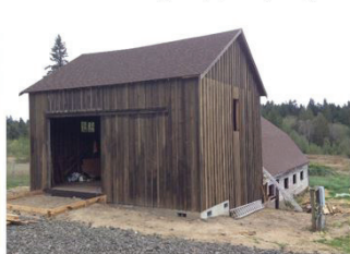
Re-construction in Progress (April 12, 2016).
