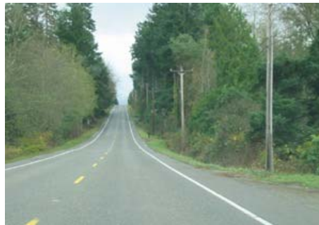
Roadside vegetation filters run-off
