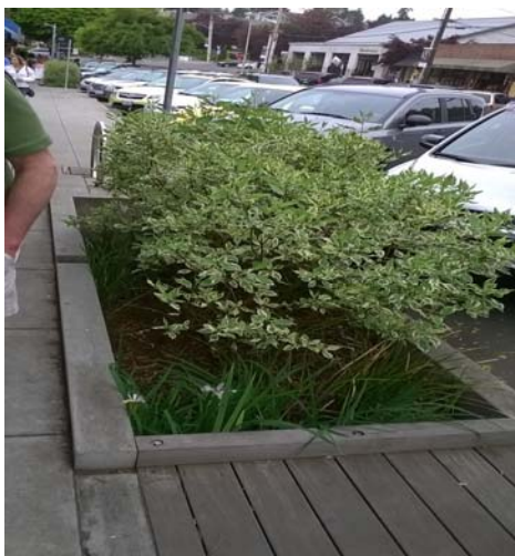
Stormwater planters to control run off and improve water quality
