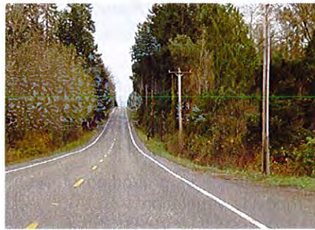
Special stormwater containment features can control water runoff roadway surfaces
