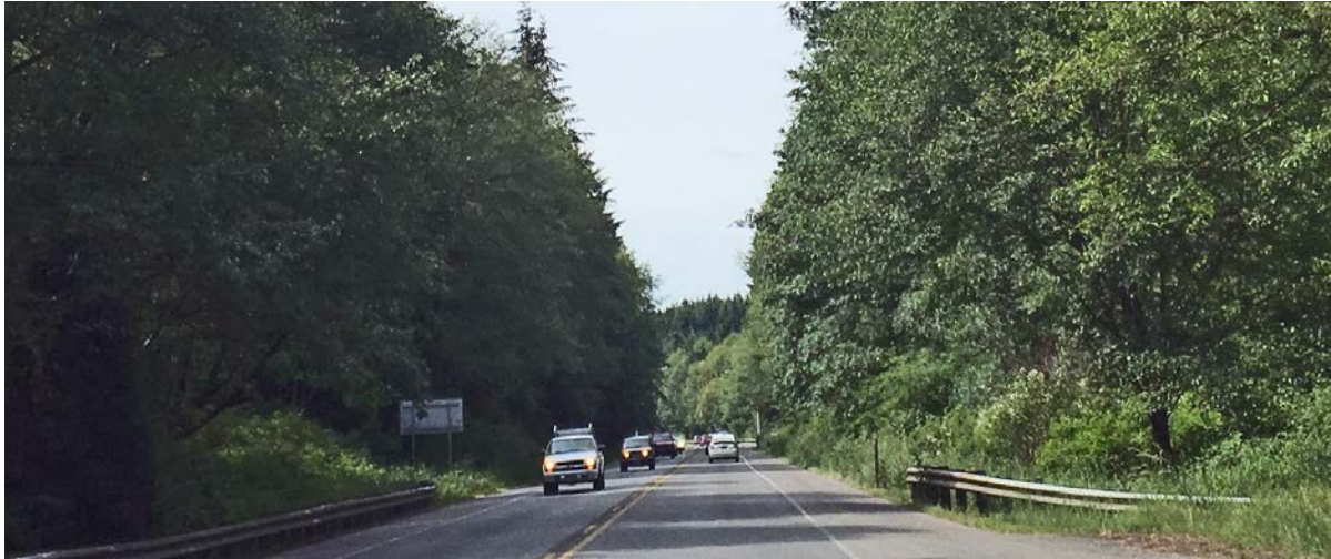
Fig. 4 The SR 305 corridor is a major part of the Island's functional mobility and visual character
