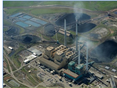
Colstrip Generating Station, MT
