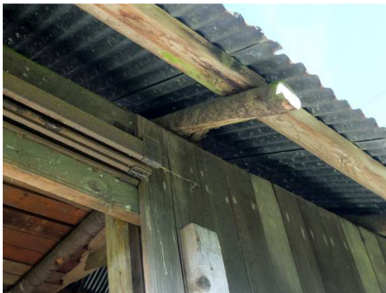
Fig.9d. Pole rafters and corrugated roof.
