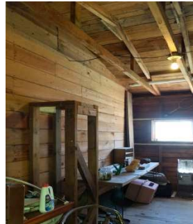
Fig. 11b. Office area.
