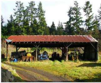
West elevation of Shed 2
