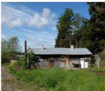
East elevation of bunkhouse
