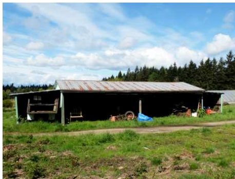
West elevation of Shed 1
