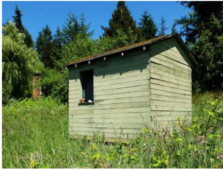
Southwest elevation of shower shed
