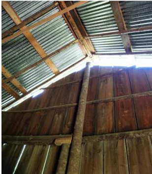
Fig.9a. Gap at ridge.
