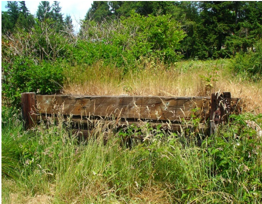
Fig. 16a. Suyematsu loading dock.
