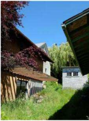
South elevation of house
