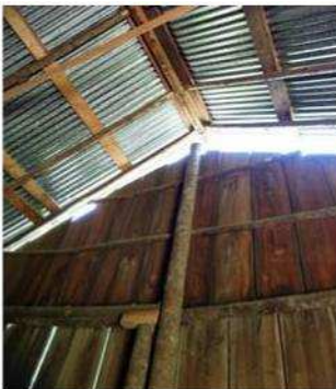
Wall & ceiling of barn
