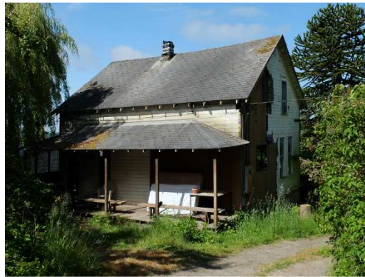
Fig. 8b. NW elevation with mixed siding.
