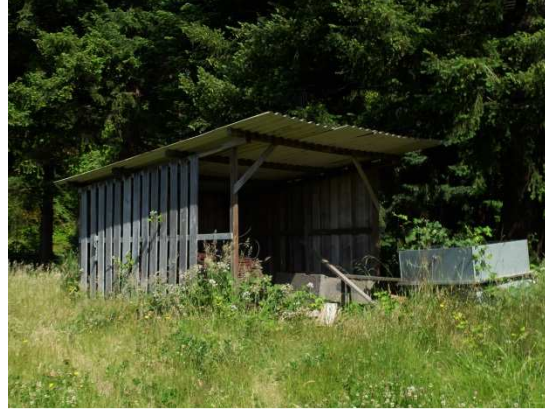
Fig. 26. SW elevation. No.26.
