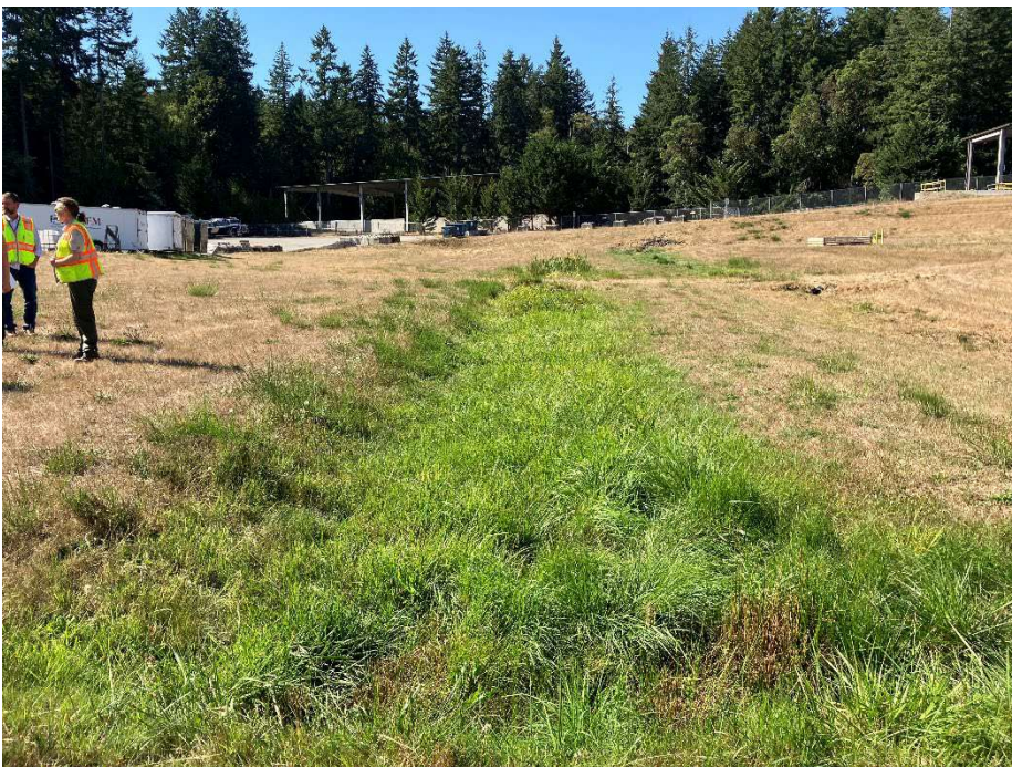
Photo [14] Description: Bio-filtration Swale down stream of sand filter.
