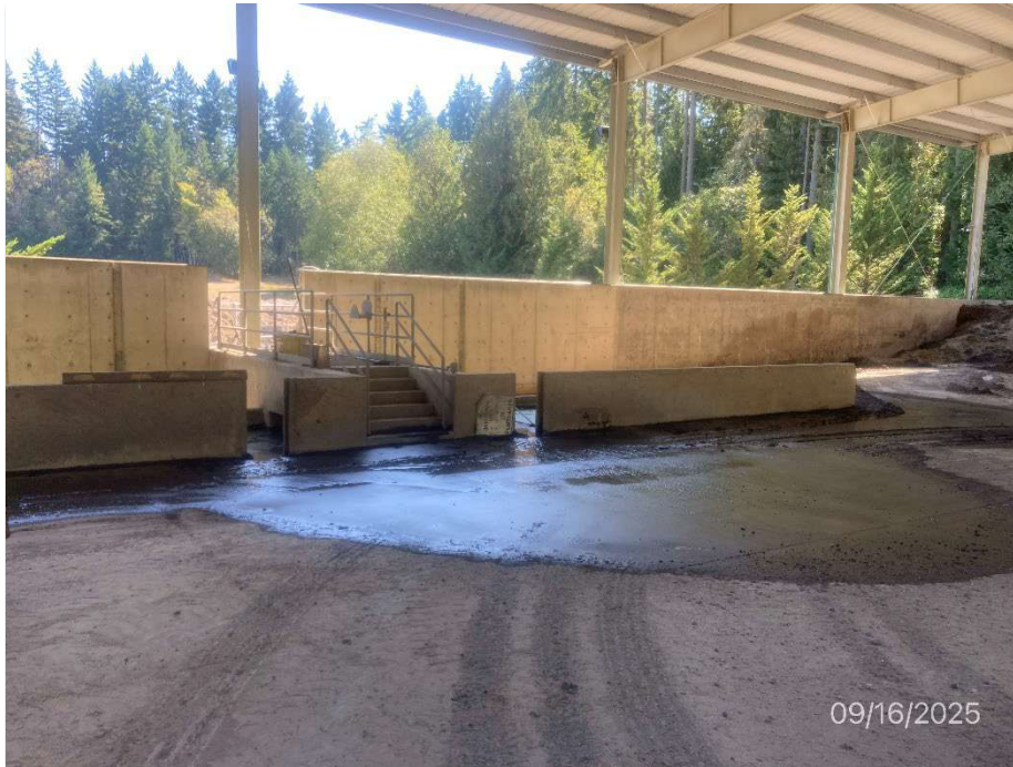
Photo [3] Description: Decant tipping floor.
