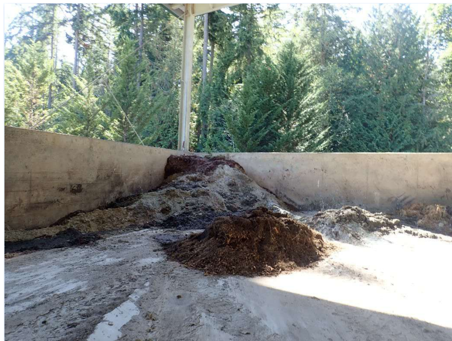
Photo [2] Description: Street waste solids storage and drying, right side of facility.
