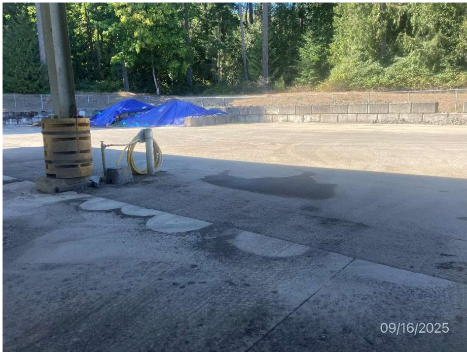
Photo [8] Description: Evidence of track out leaving the decant facility to rest of yard. Moisture on ground was due to street sweeper filling up water tank
