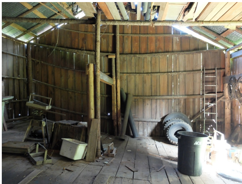
Interior view of barn facing north (2014).
