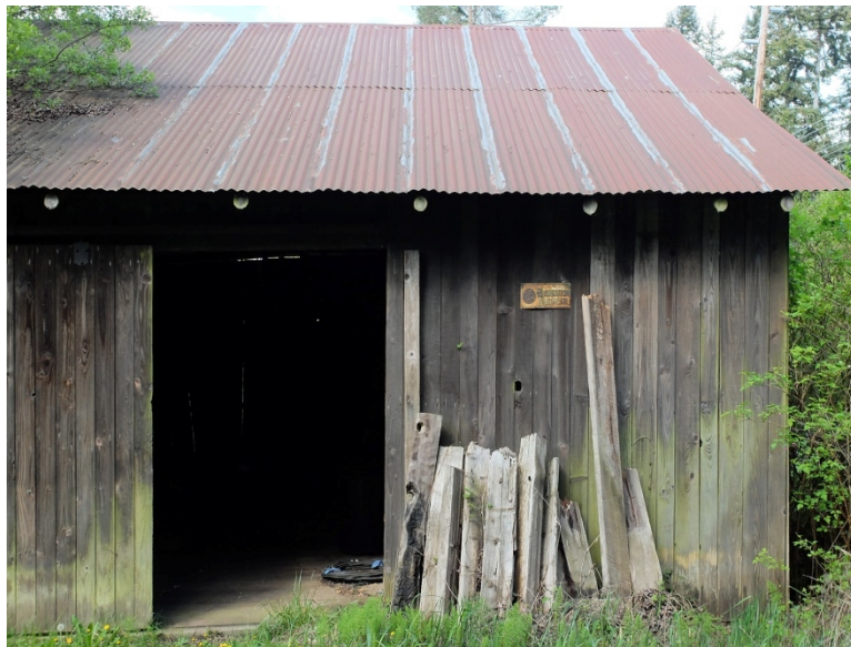
East elevation of barn (2014).
