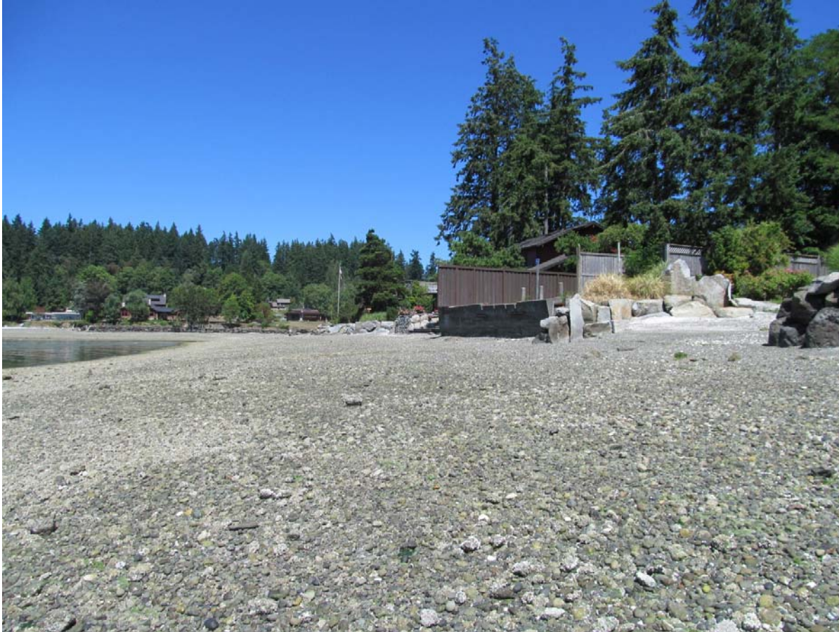
Figure 2. Photo of the project site looking north. The water is on the left and the seawall on the right. The top layer of the beach generally consists of very coarse to coarse gravel.
