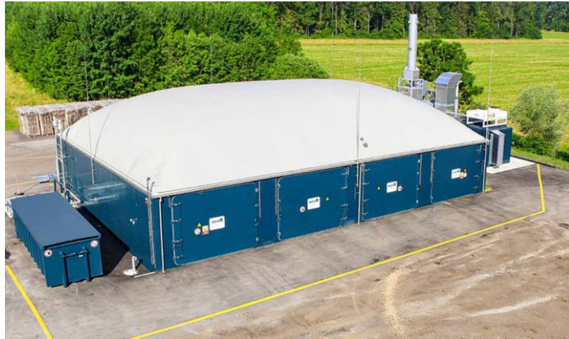
Figure 9. Small plant digester system. Picture from Bekon.
