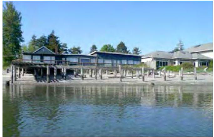
Removing unused piers can provide shoreline mitigation.
