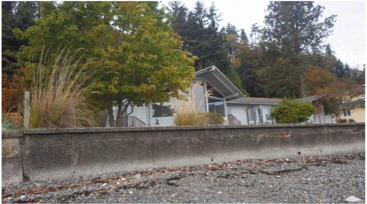
BULKHEAD; SOUTHERN PROPERTY LINE
