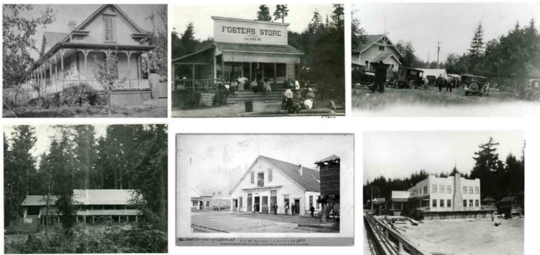
Figure 3. Historic Images of Island Center
