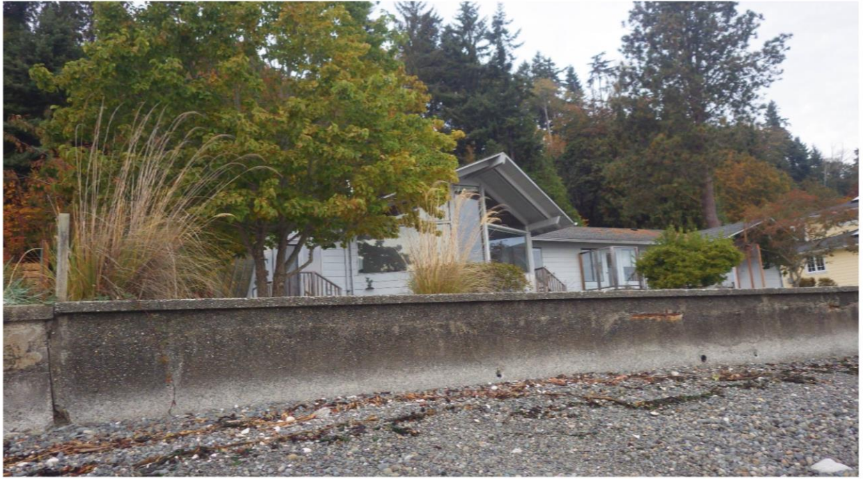
BULKHEAD; SOUTHERN PROPERTY LINE
