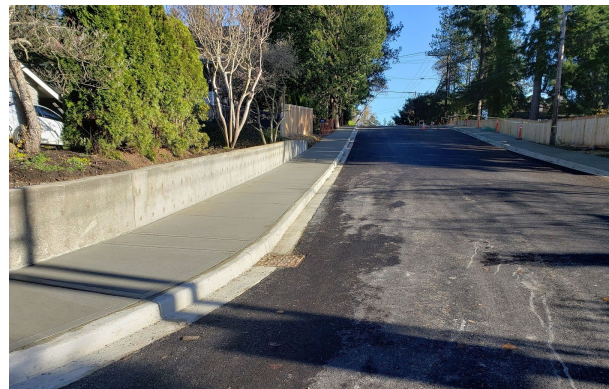
Complete street, water main, and storm drainage improvements on Wyatt Way (COBI)
