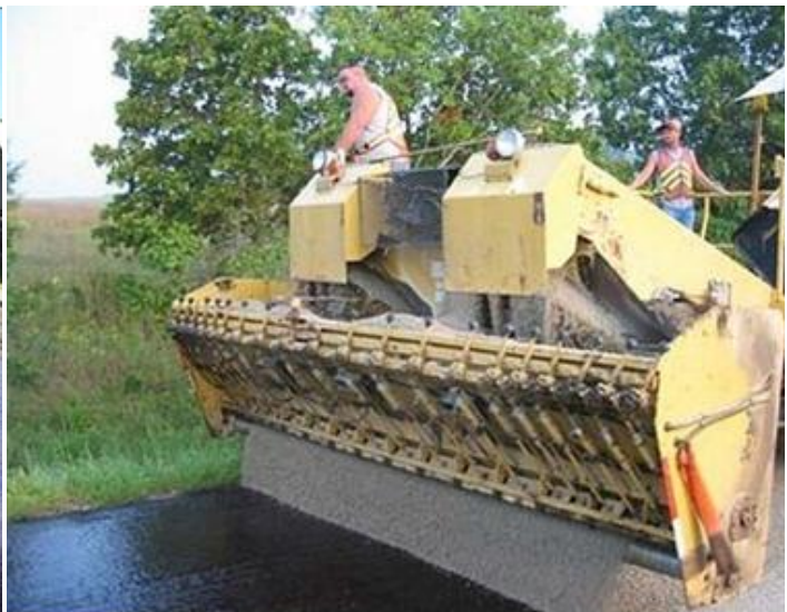
Crushed rock is spread over the emulsified asphalt oil and then rolled to embed the rock into the oil.
