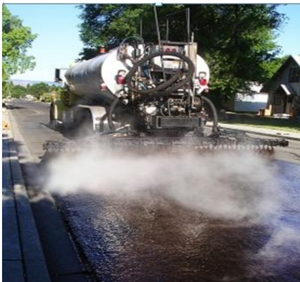
Oil emulsion is applied to the road surface
