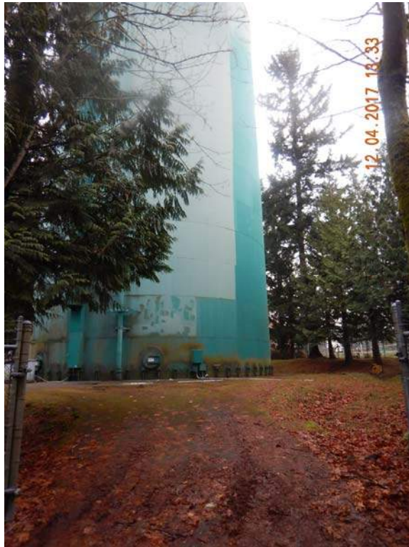
Plate 1 – Existing 1.5 MG reservoir.
