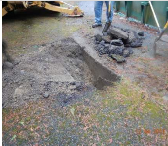
Plate 2 – 1.5 MG reservoir foundation approx. 3 feet thick at TP-2.
