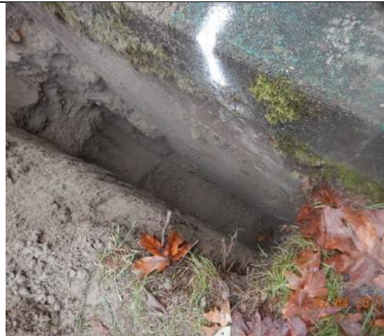
Plate 3 – 1.0 MG reservoir foundation approx. 10 feet thick at TP-4.
