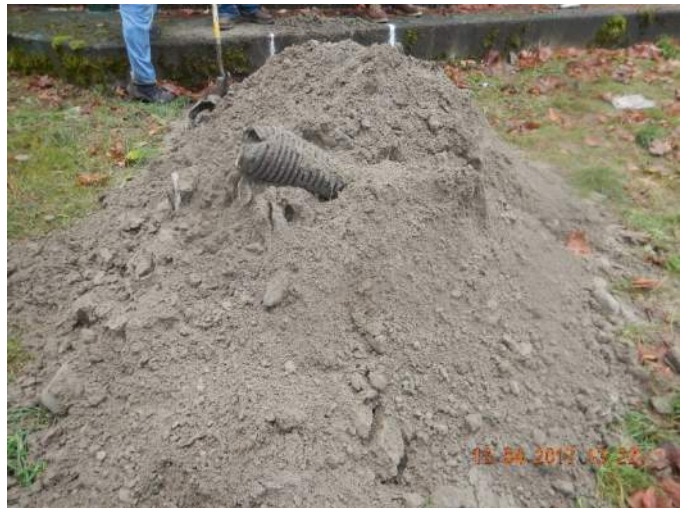
Photo TP-4B: View of Test Pit TP-4 excavation spoils
