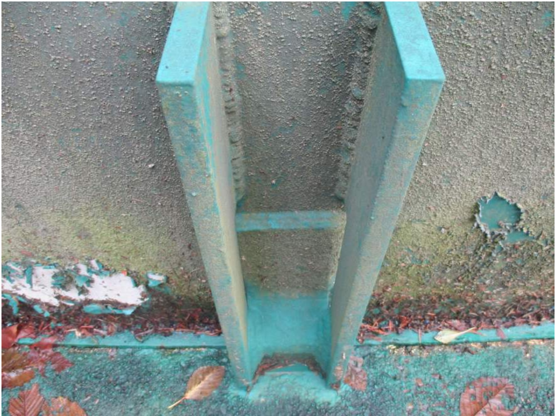
B: SEISMIC STRAPS
