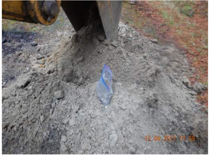
Photo TP-2B: View of Test Pit TP-2 excavation spoils.
