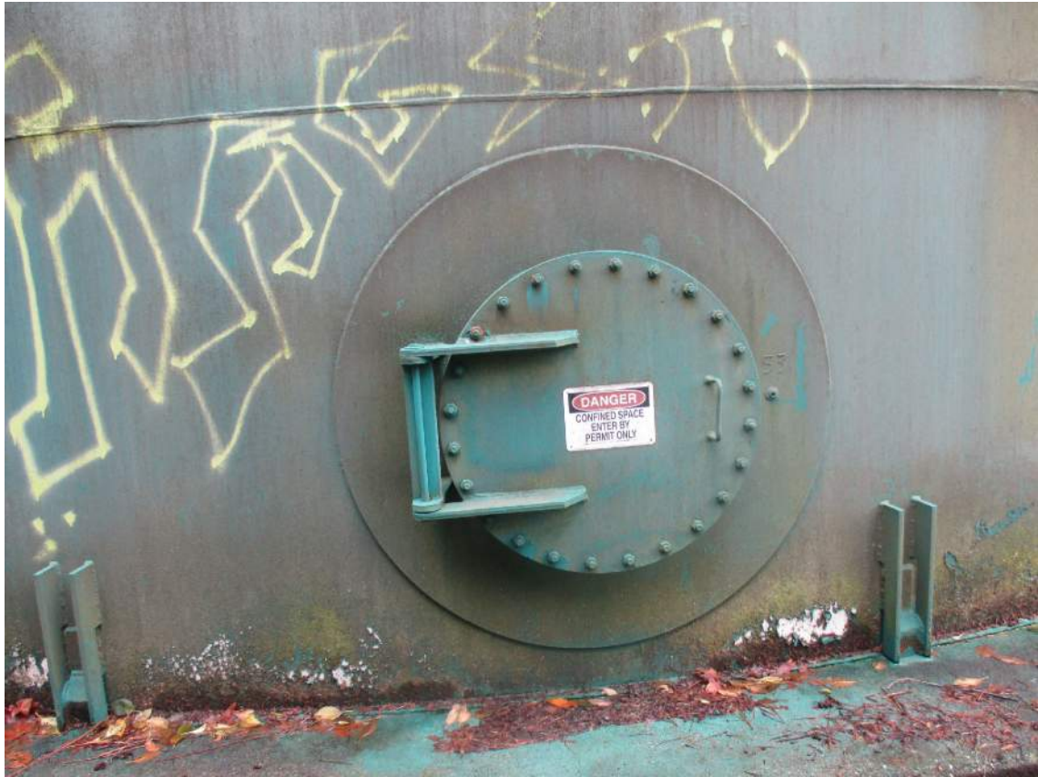
A: EXISTING 30-INCH MANWAY
