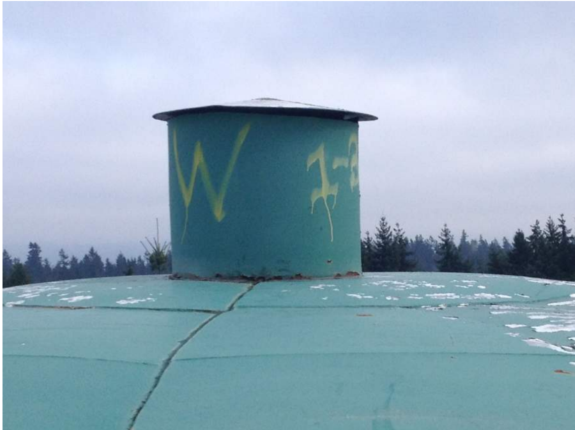
C: RESERVOIR ROOF VENT
