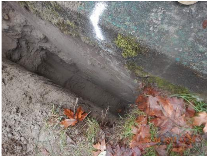
Photo TP-4A: View of Test Pit TP-4 at 10 feet deep. Reservoir foundation is exposed on the side of test pit.
