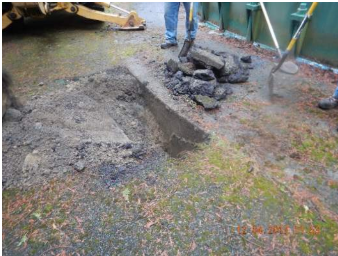
Photo TP-2A: View of Test Pit TP-2 at 3 feet deep. Reservoir foundation is exposed.
