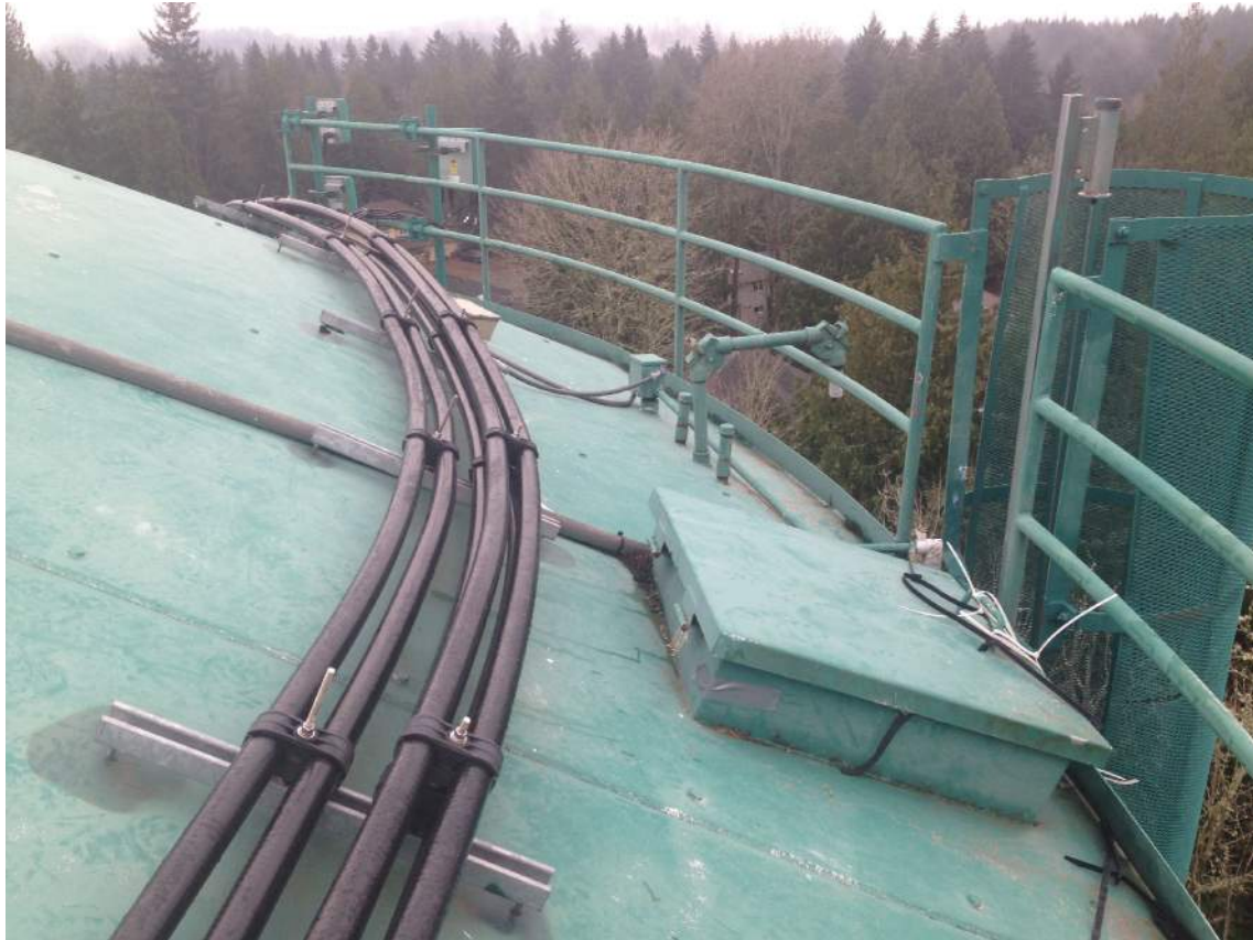
C: RESERVOIR ROOF INCLUDING ROOF ACCESS HATCH
