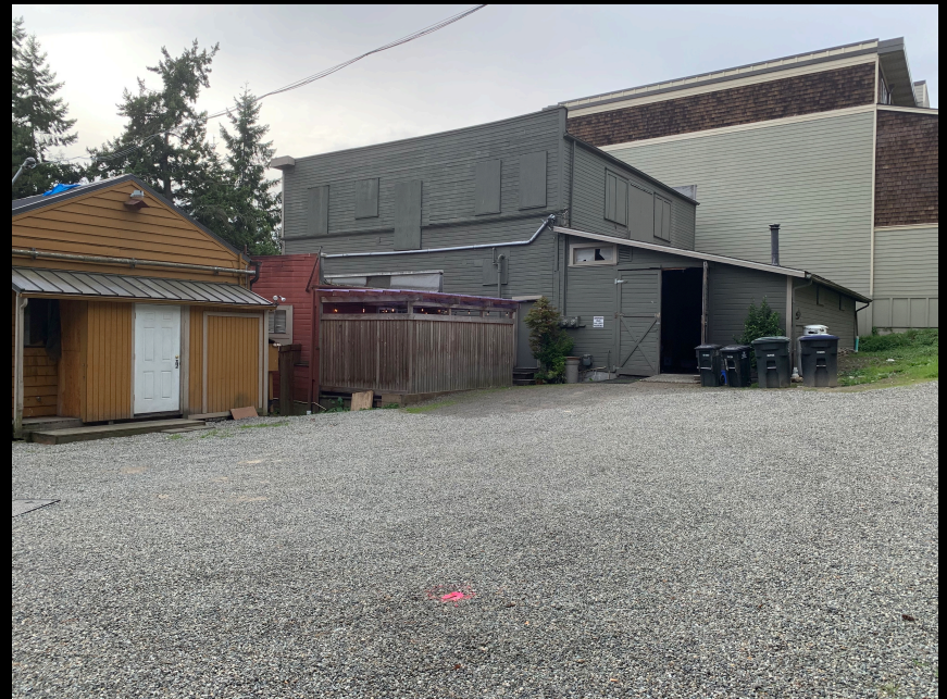
Back of existing buildings
