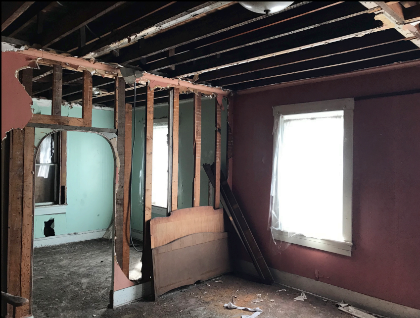
Existing condition at second floor
