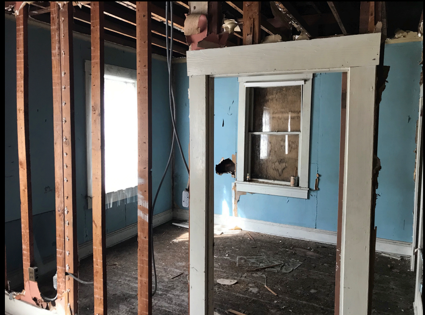
Existing condition at second floor
