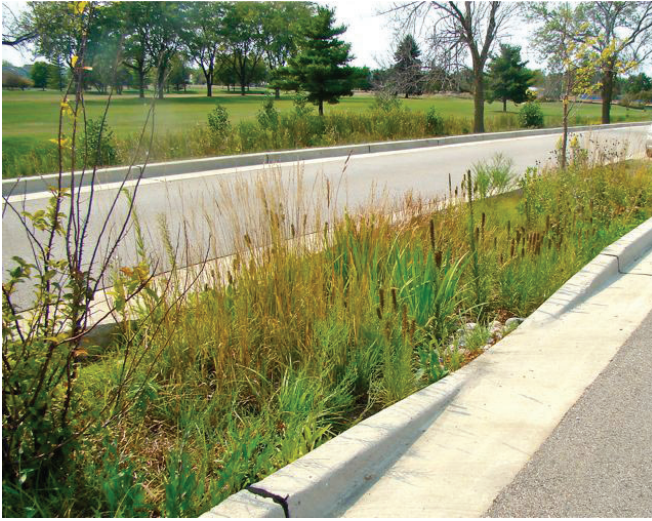
Vegetated median strips or splitter islands
