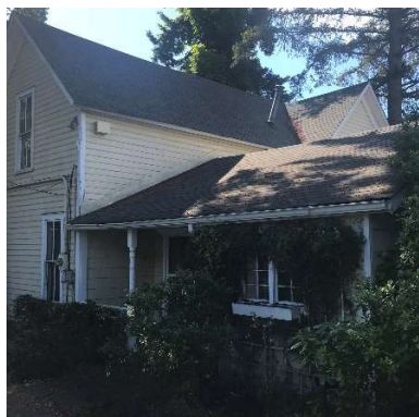
Photo of North Entry
