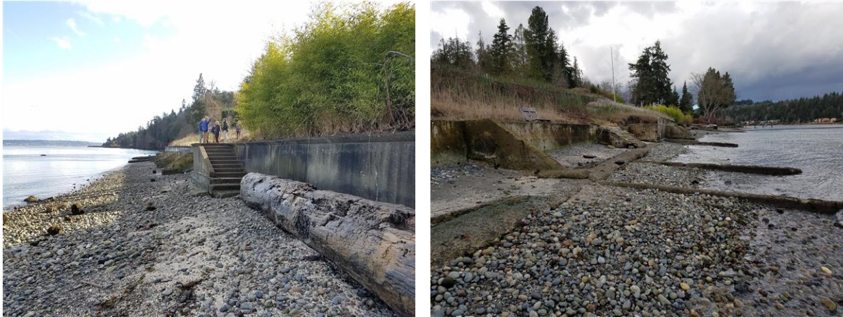
Figure 2. Existing bulkhead looking west (left) and east (right)
