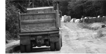
Trees cut in State Route 305 Scenic Byway due to city using federal grants for STO Trail.
