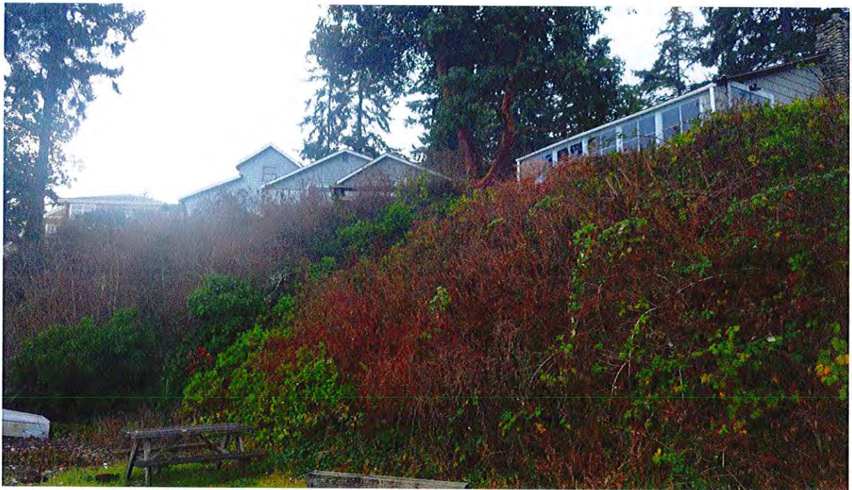
SLOPE FACE. STRUCTURE ABOVE
