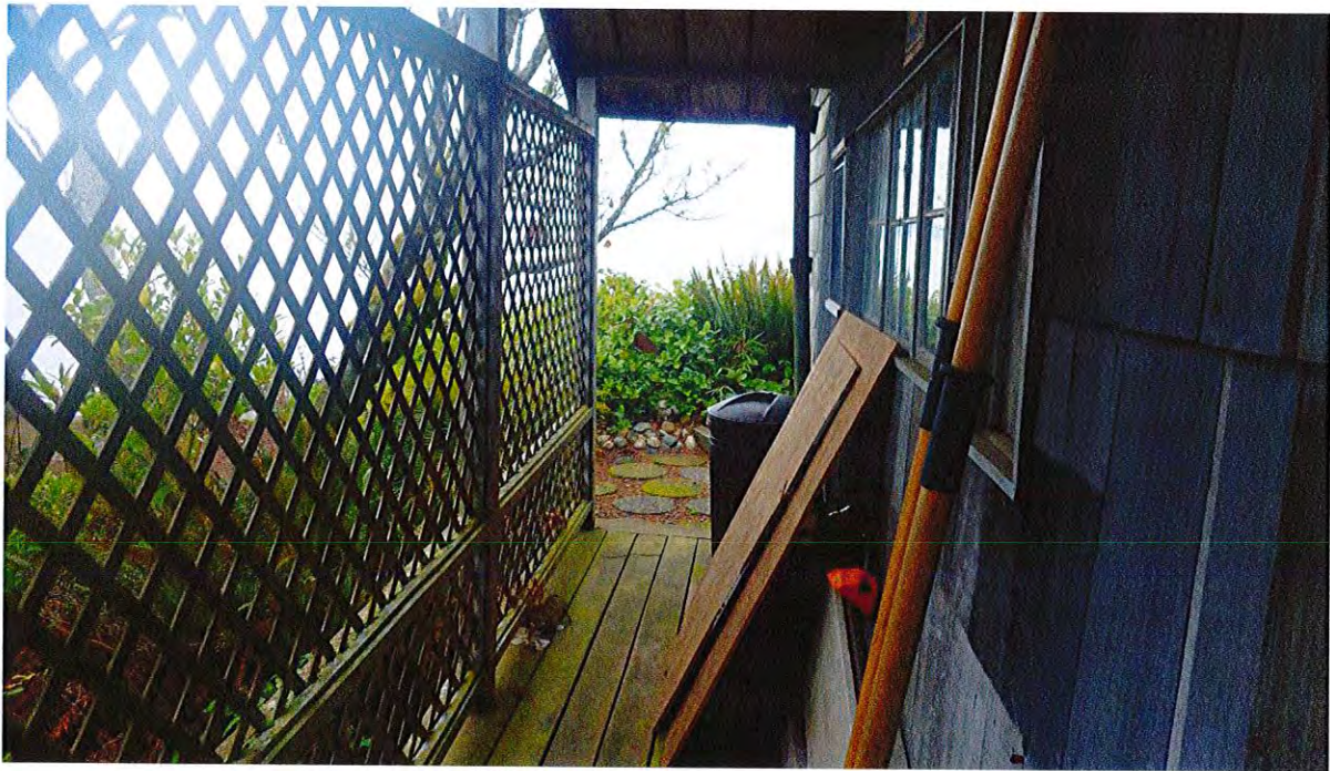
DECK ALONG THE NORTHERN SIDE OF STRUCTURE (COVERED)
