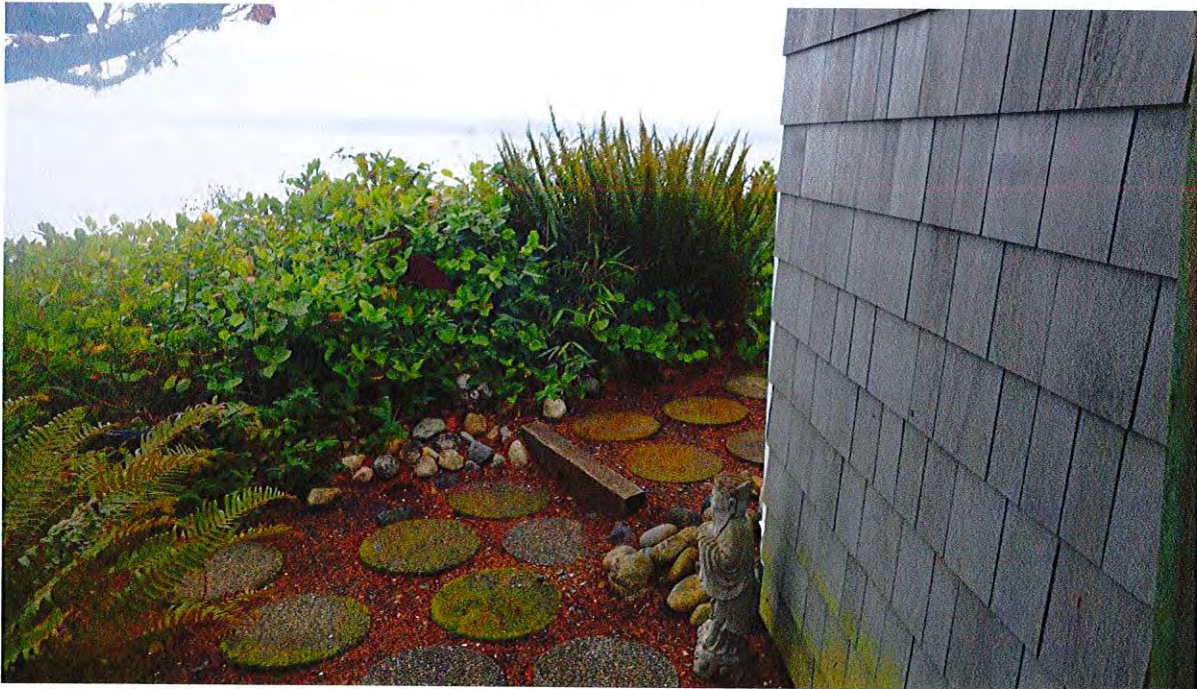
ACCESS ALONG FRONT OF STRUCTURE AND TOP-OF-SLOPE
