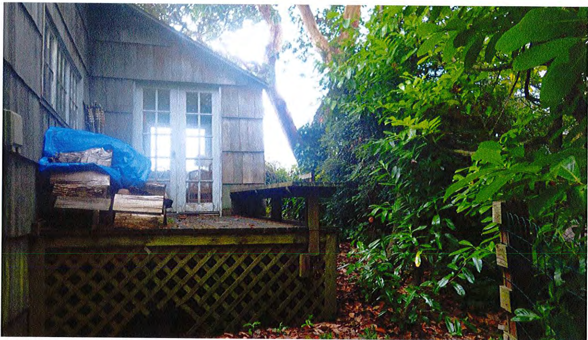
DECK ALONG SOUTHERN SIDE OF STRUCTURE
