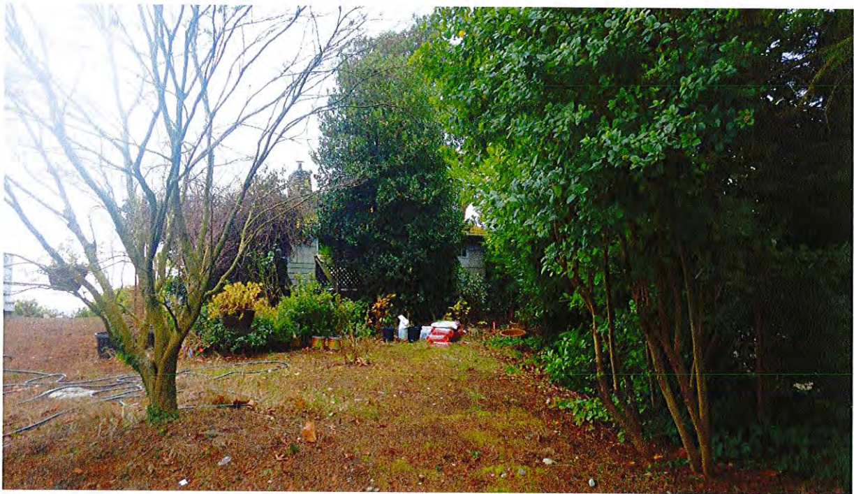
ENTRY TO EXISTING STRUCTURE
