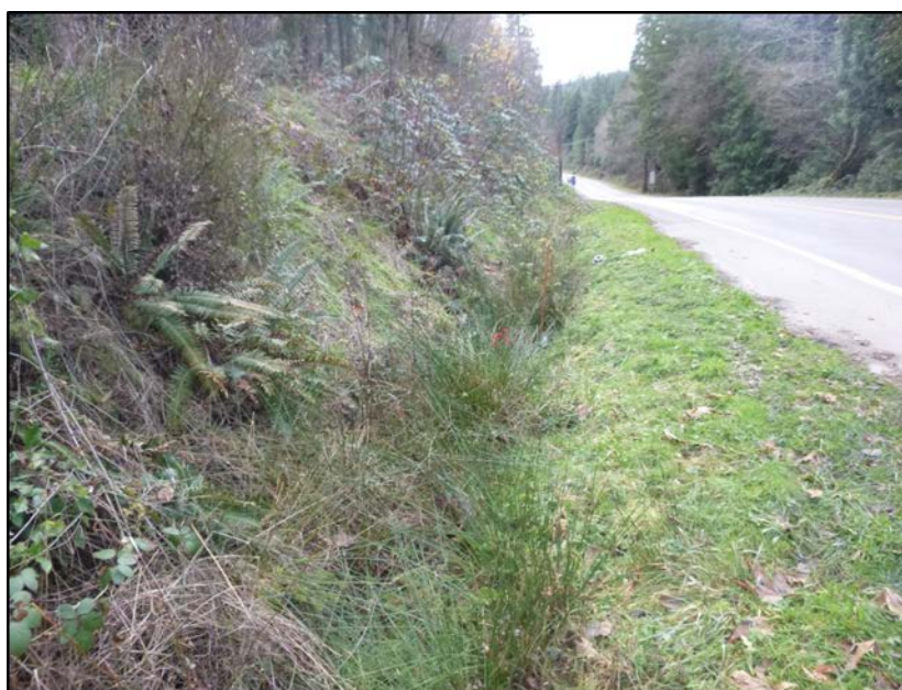
Drainage ditch west of the Suzuki Property
