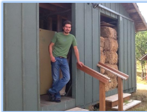
New steps and railings were constructed
